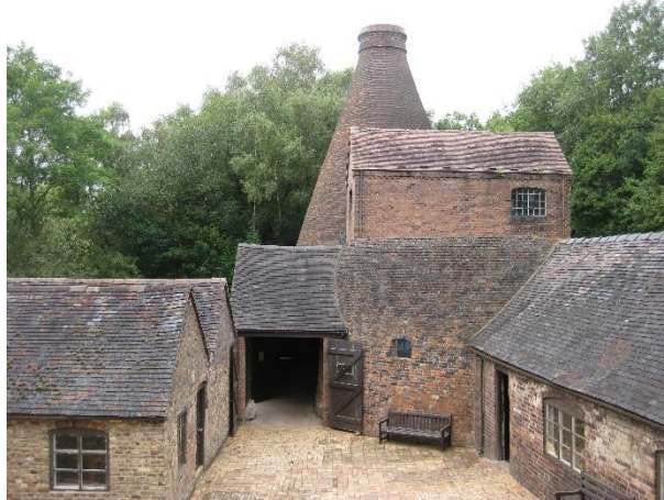
The same kiln with some of the factory buildings.
