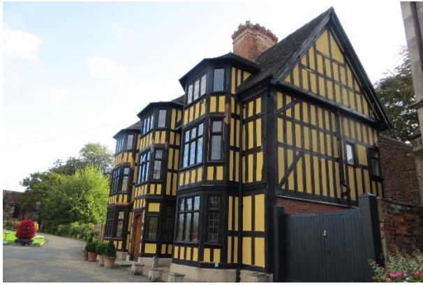
The bright Castle Gates House. On the left is the entrance to the castle.
