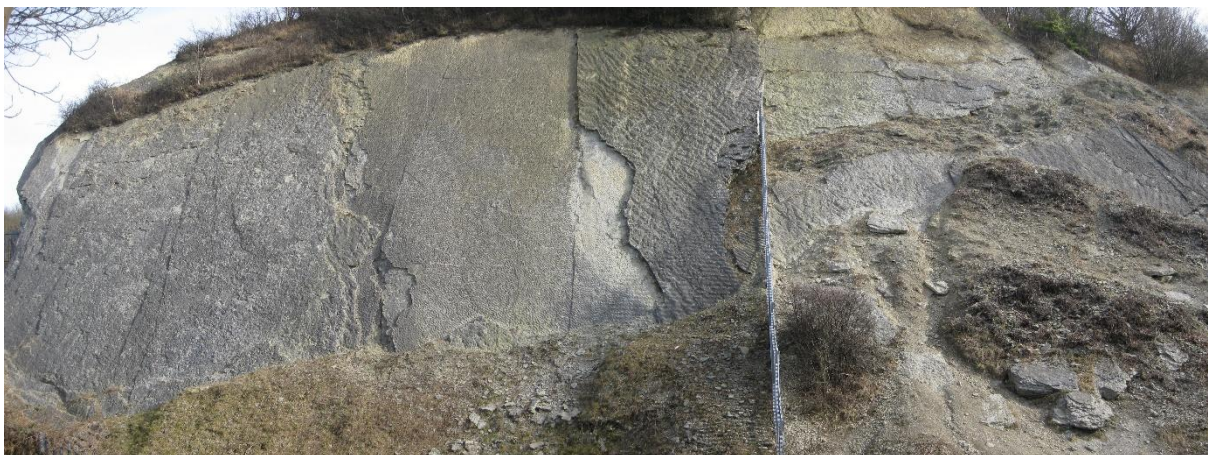
A section of the rock face. The apparent vertical join is a metal fence. Why? Who knows.
