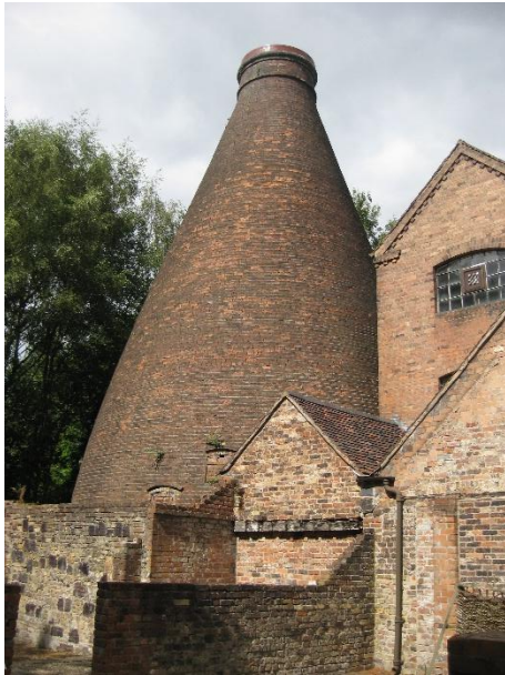
A remaining kiln.
