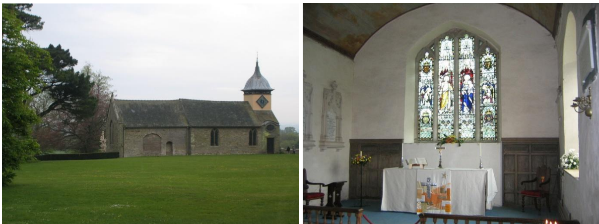
Church of St Michael and stained-glass window.
