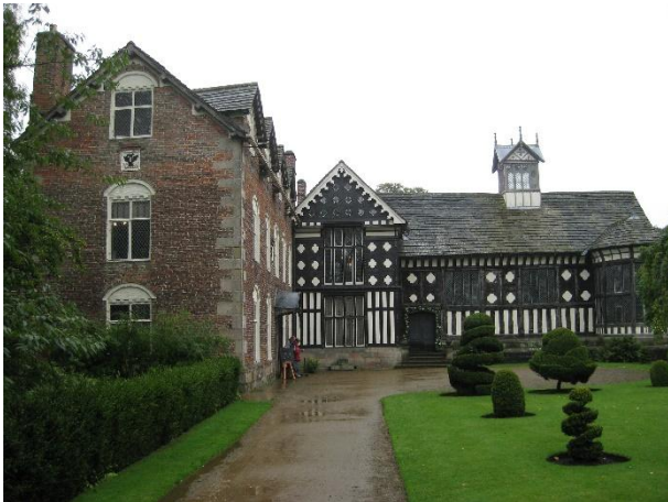
The older Great Hall on the right. The lantern tower was added in 1825. The newer 1662 brick building on the left.
