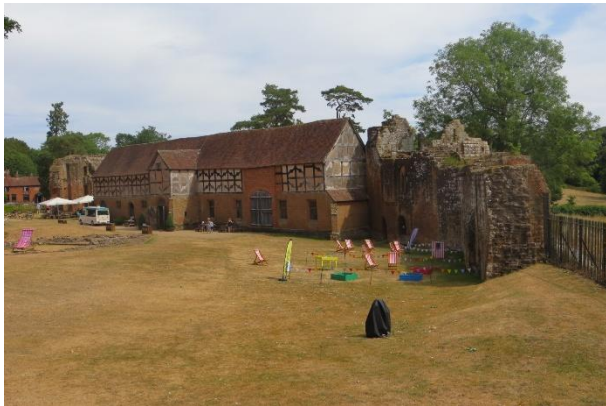
The Stables with the Water Tower in the foreground.
