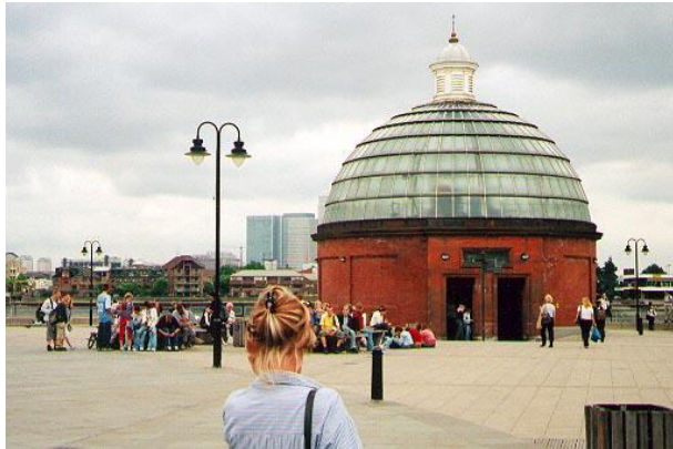
The Thames Foot Tunnel at Greenwich.
