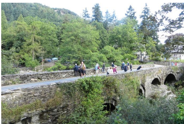
The Pont-y-Pair bridge.
