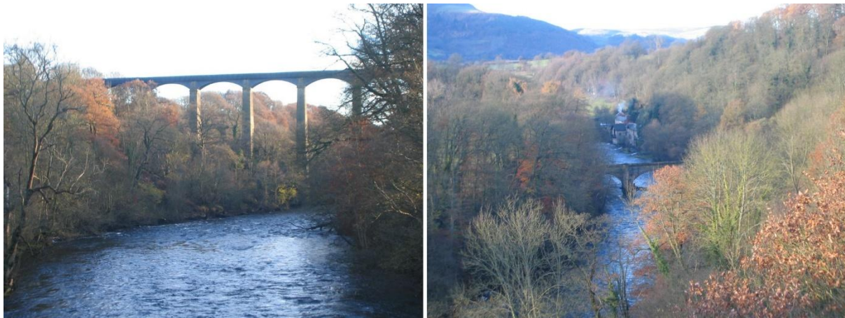
Pontcysyllte canal aqueduct seen in winter sun from the road bridge and looking down the valley from the aqueduct to the road bridge.
