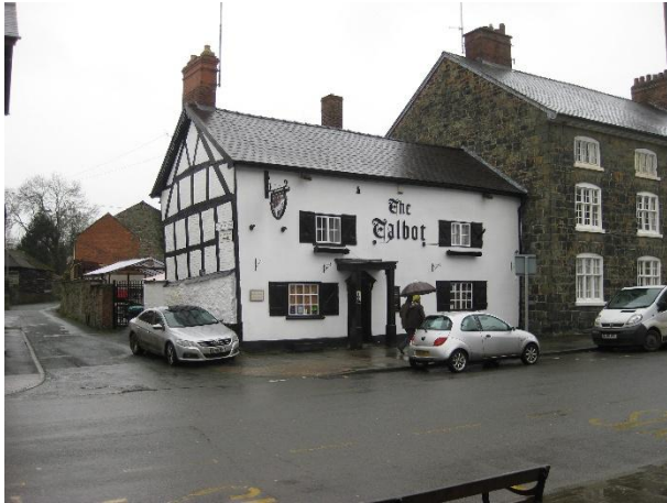
The 16 th century timber frame Talbot Inn.
