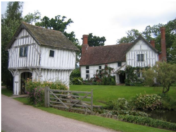
Lower Brockhampton gatehouse & manor.
