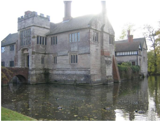
Baddesley Clinton showing part of the moat and the main entrance on the left.
