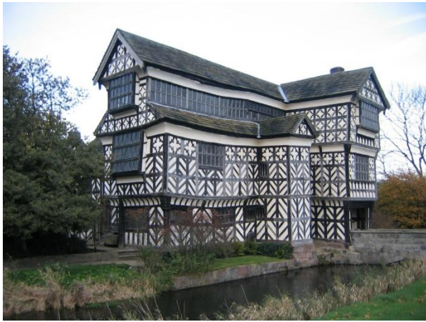
Little Moreton Hall Gatehouse south range.
