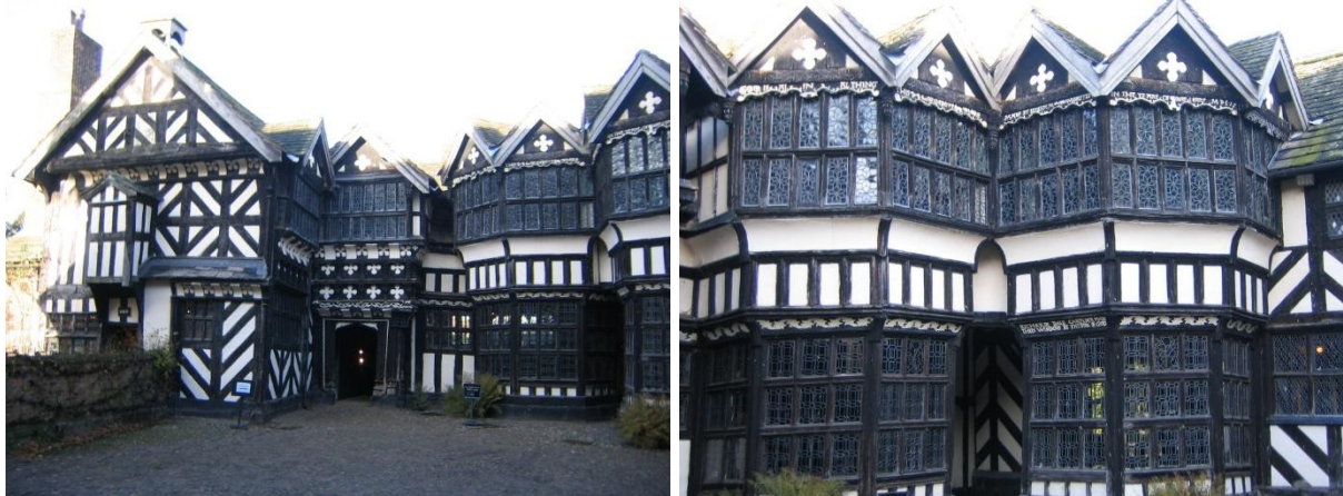
In the courtyard looking north at the Great Hall with the bay windows on the right.
