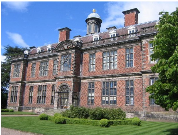
Sudbury Hall. Notice the unusual brick cross hatch pattern.
