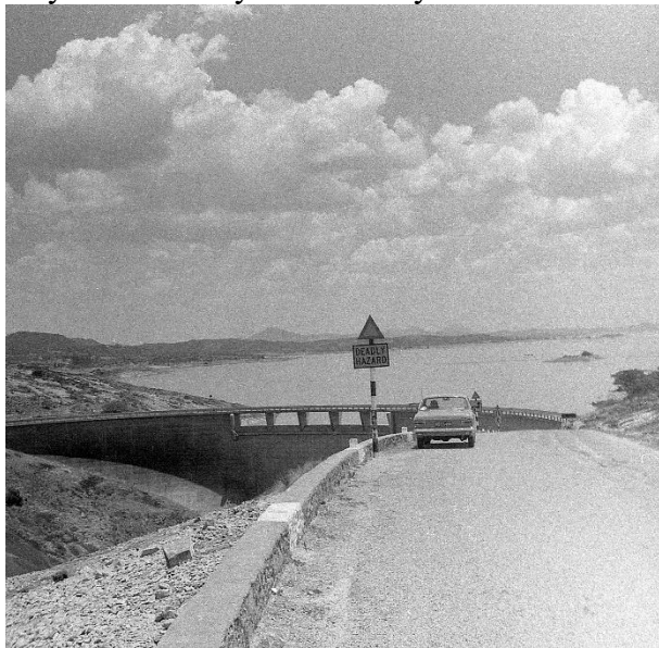
Kariba Dam with Ford Escort ND 155 466 in the foreground.
