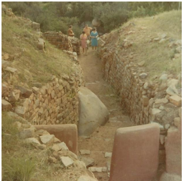
The size of the dry-stone walls, that is no use of mortar, were increased with time. Newest
