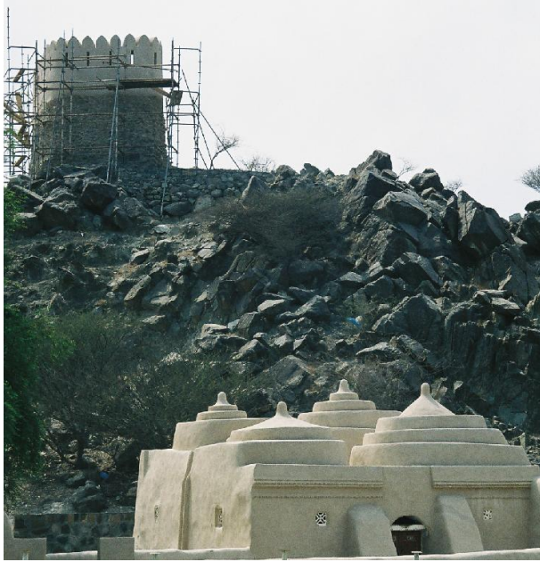
Bidiya Mosque circa 640 with one of the watchtowers undergoing restoration.
