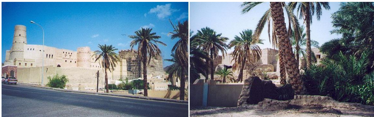
Bahla Fort partly restored and a date palm garden.
