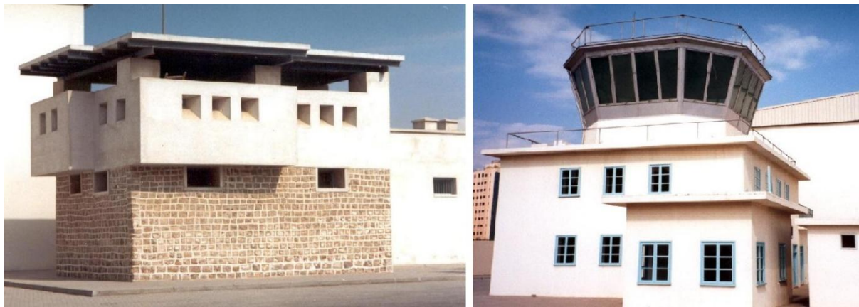
The restored fort/hotel and control tower building.
