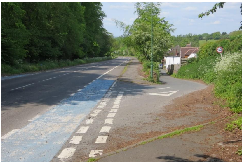
Downhill view of the Birmingham Road embankment and steeper Old Road to the right. The Queen's Head is hidden off to the distant right where the road begins to curve to the left.
