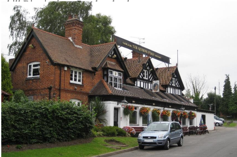
The Queen's Head pub at Old Road level. Notice the different west wall from the east wall seen above.
