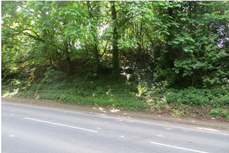
Meriden Hill. The cutting depth at the top is evident by sky/ground discontinuity between the trees.
