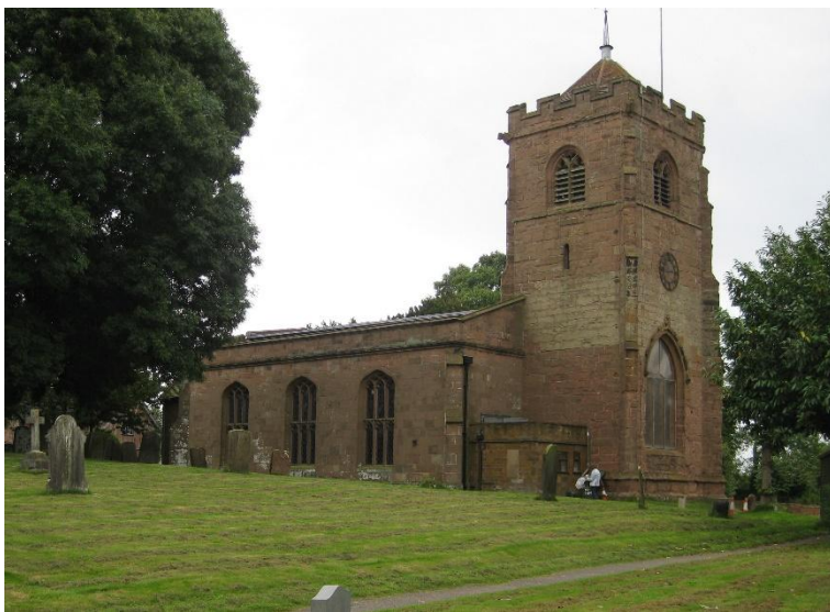
St Laurence Church seen from the north-north-east.
