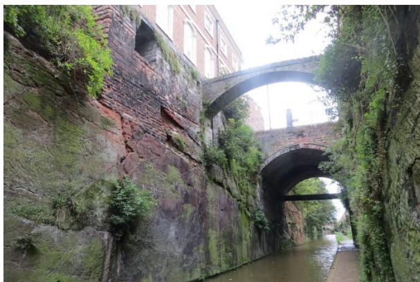
Northgate seen from the canal towpath looking east. Beneath it is a waterpipe. In the foreground is the Bridge of Sighs.
