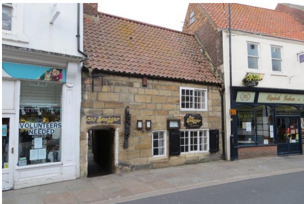
The small entrance in Baxtergate Road.
