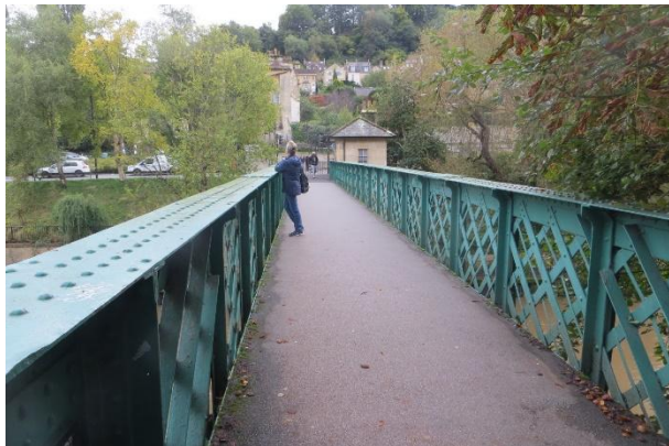
The Half Penny Bridge and toll building.
