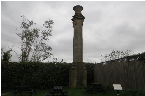
The Bathwick Hill pump house chimney.
